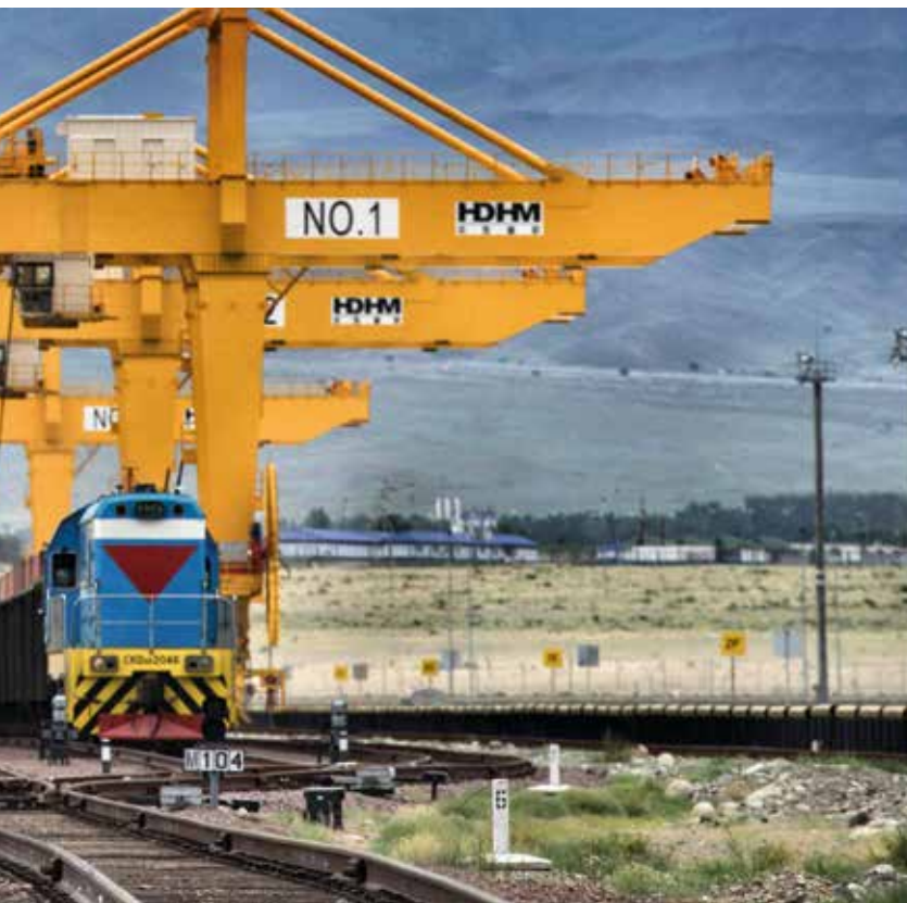
Rail terminus at Khorgos Gateway. Containers are transferred from Chinese to Kazakh trains at Khorgos, due to different track gauges.
