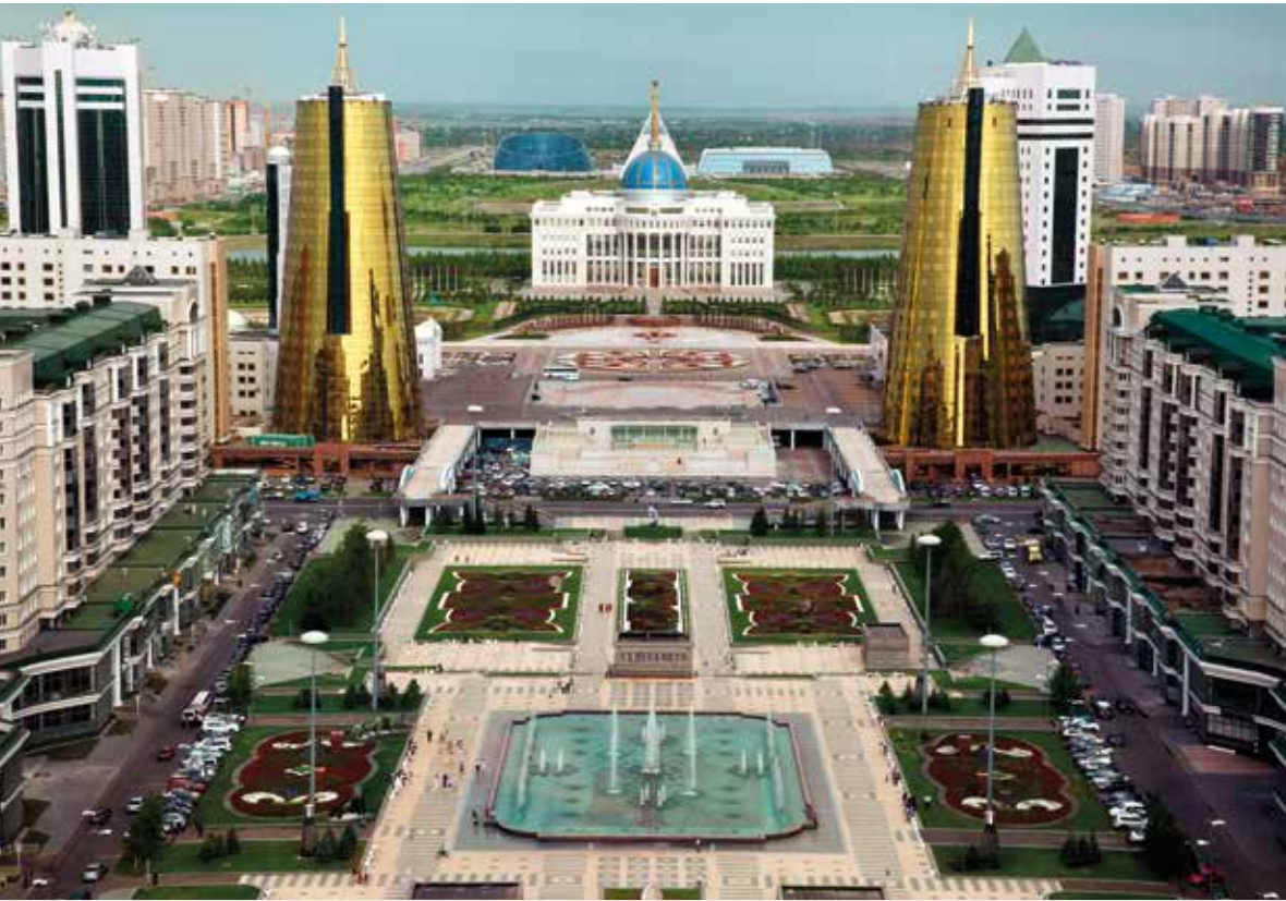
4. Golden tower of the House of Ministries and its main plaza. Architects: Shokhan Mataibekov, Zhexen Aynabekov, and Rafik Musabayev. Photo credit: Ryan Koopmans.
