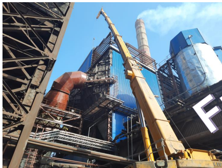
ESP Filter installation at Sinter Plant - 5
